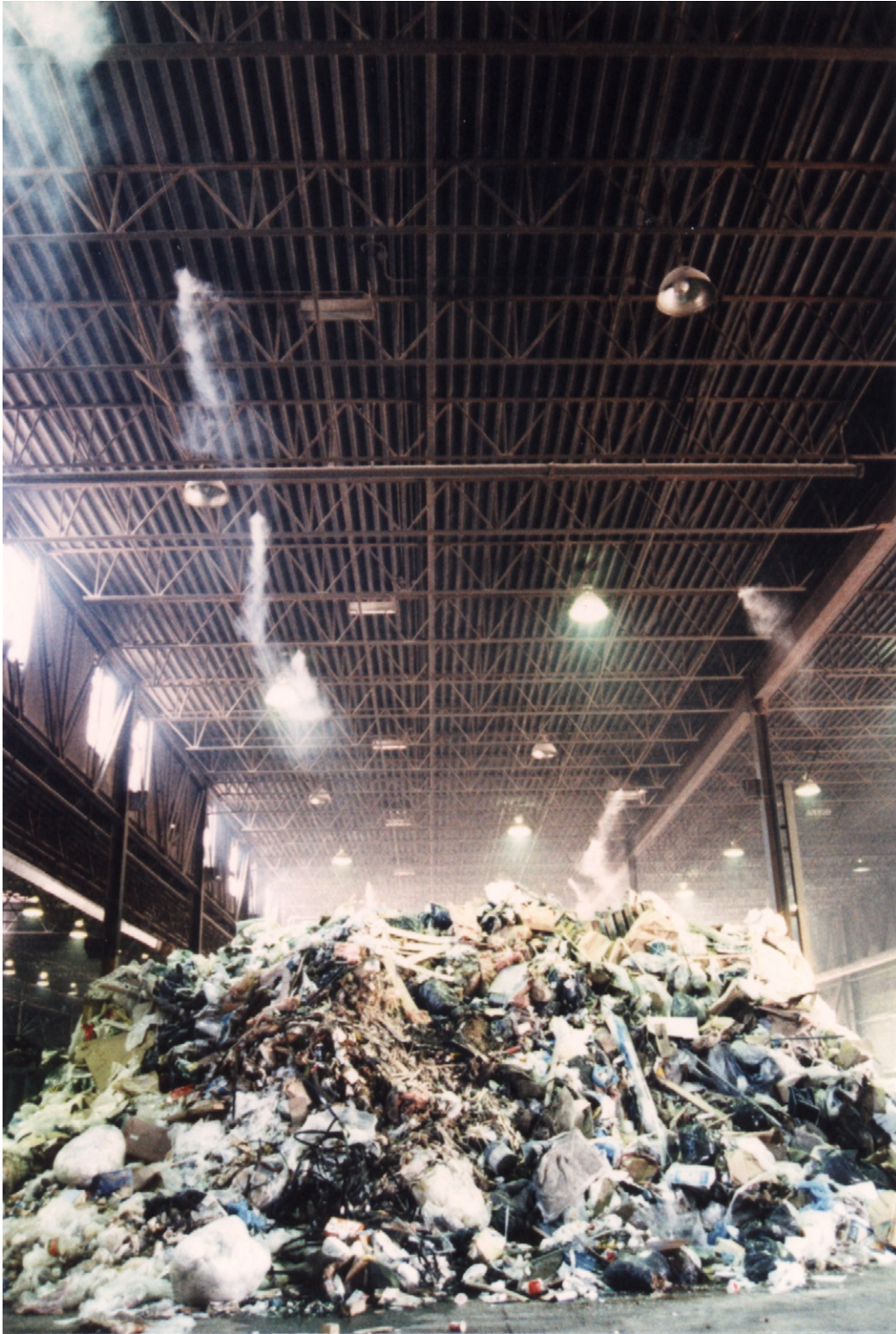
Overhead nozzles at a garbage transfer station.
